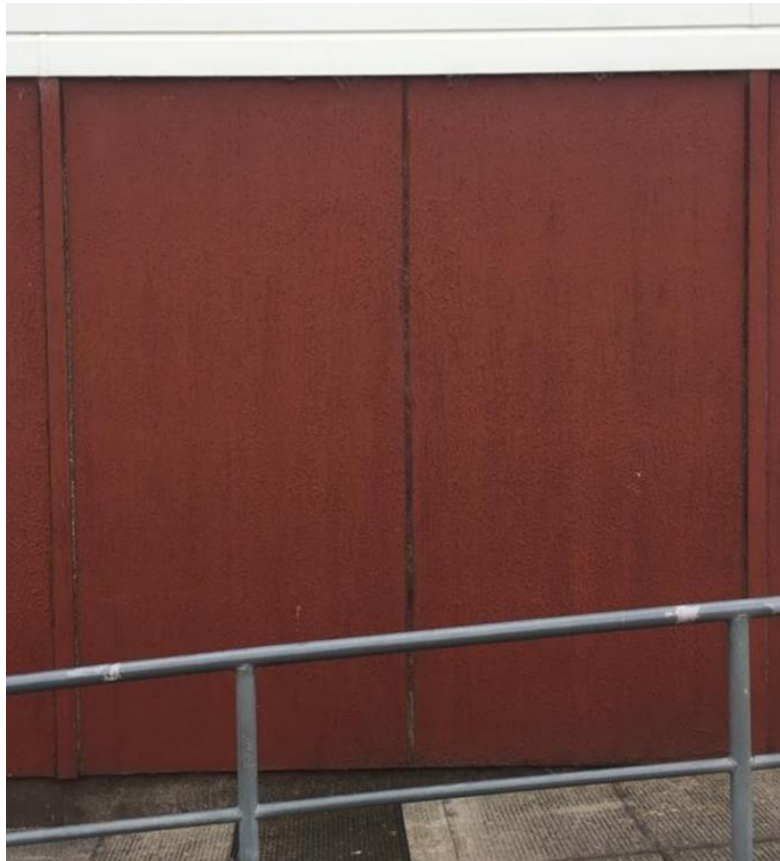
Back wall of mobile classroom on junior playground before.
