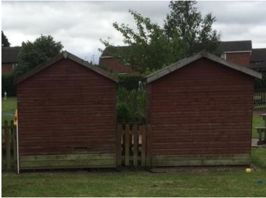
Sheds at the back of the mobile classroom before.
